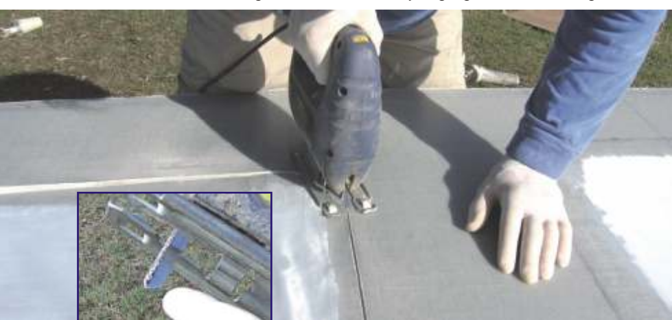
Then a jig saw for the curves. I found a great tool bit for cutting composite panels. See inset; it's carbide sintered, no teeth. The abrasive grit doesn't show any wear so far.
