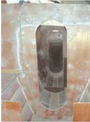
Bulkheads in hull
